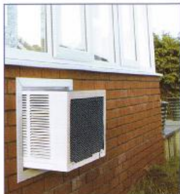
View of Debonair unit from exterior
